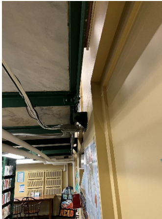
Photo 3 – Floor system at stacks supported at exterior wall
