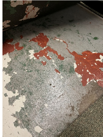
Photo 8 – Buckling in subfloor
