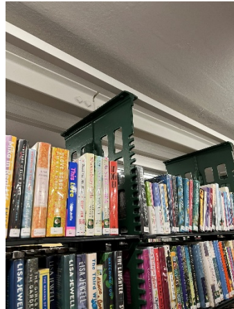
Photo 2 – Structural shelving system supporting floor
