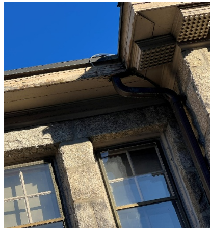
Photo 6 – Failed Gutter
